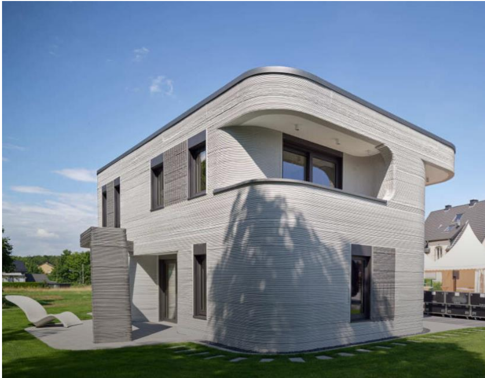
Figure S116. Picture of the house 3D-printed in Germany. Retrieved from 3D Printed House By Mense Korte Architekten & PERI 3D Construction (parametric-architecture.com) .
