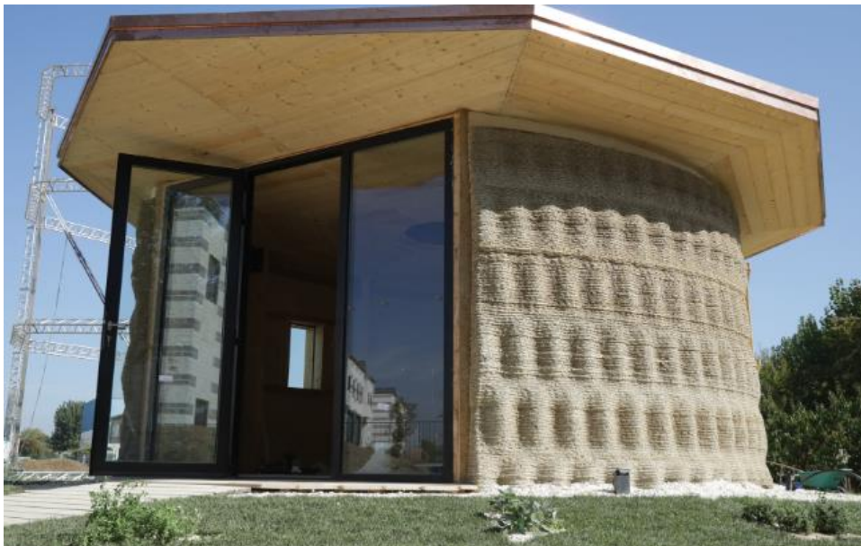
Figure SI18. Picture of the house GAIA 3D-printed by WASP in Italy. Retrieved from La prima Casa Stampata in 3D generata con la Terra | Gaia - Stampanti 3D | WASP (3dwasp.com) .
